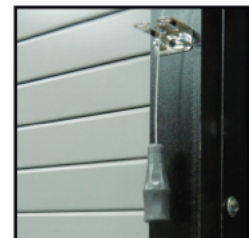
Close and Test Cable
